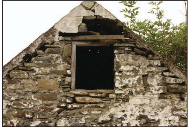
Plate 19 - Window opening northeast elevation A05
