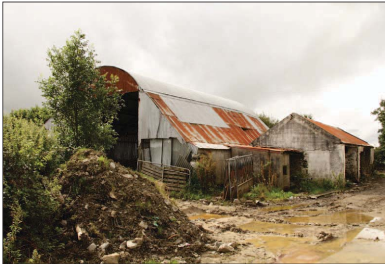
Plate 53 - North and east elevations B05
