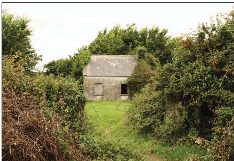
Plate 63 - Boundary wall facing north C05
