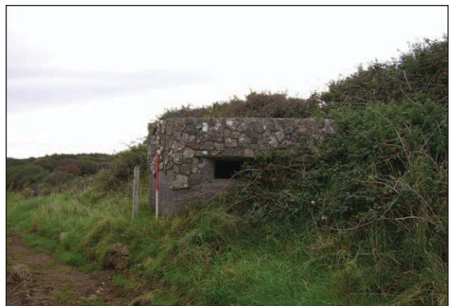
Plate 68 - Northwest elevation D01
