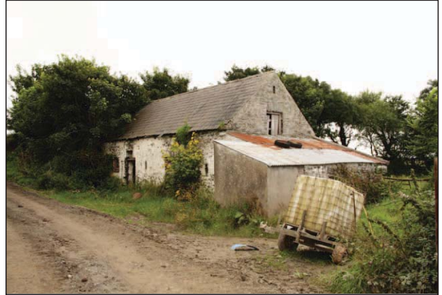
Plate 51 - East and North elevations B03
