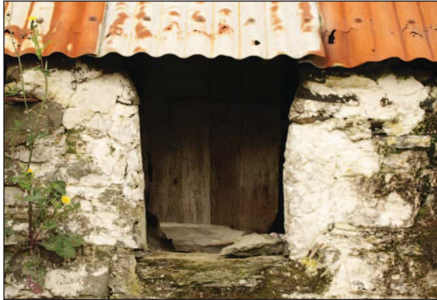
Plate 20 - Window opening southeast elevation A05
