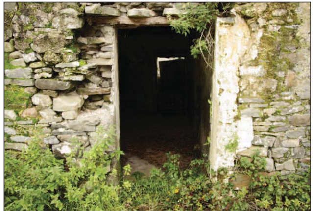
Plate 5 - Door opening southeast elevation A01
