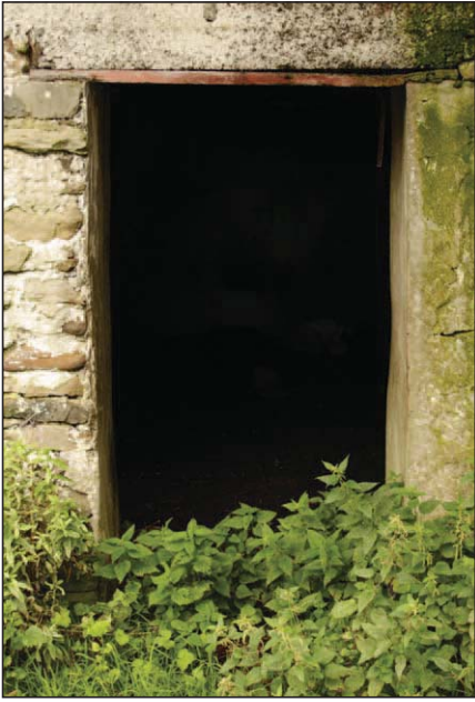
Plate 24 -Door opening southeast elevation A06
