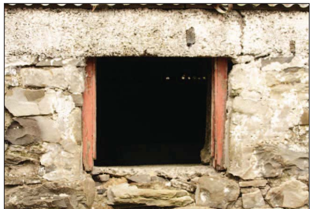
Plate 23 - Window opening southeast elevation A06_
