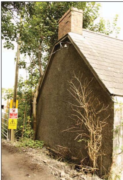
Plate 38 - West elevation B02
