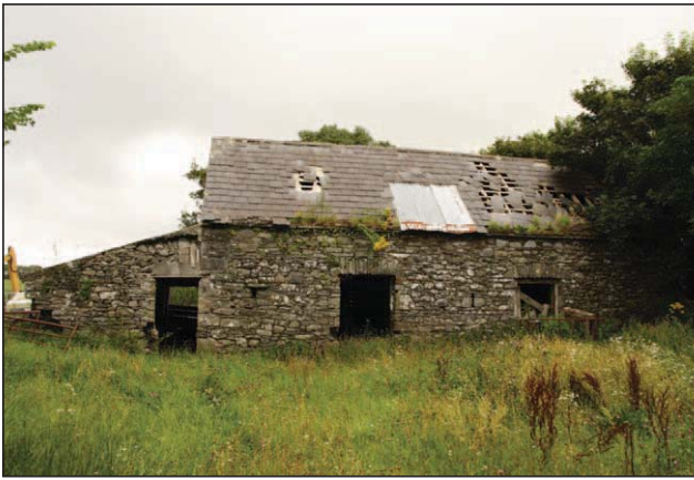
Plate 46 - West elevation B03
