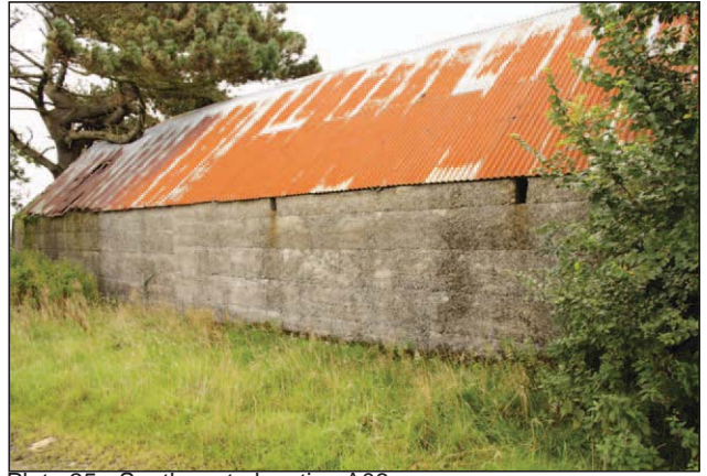
Plate 25 - Southwest elevation A06
