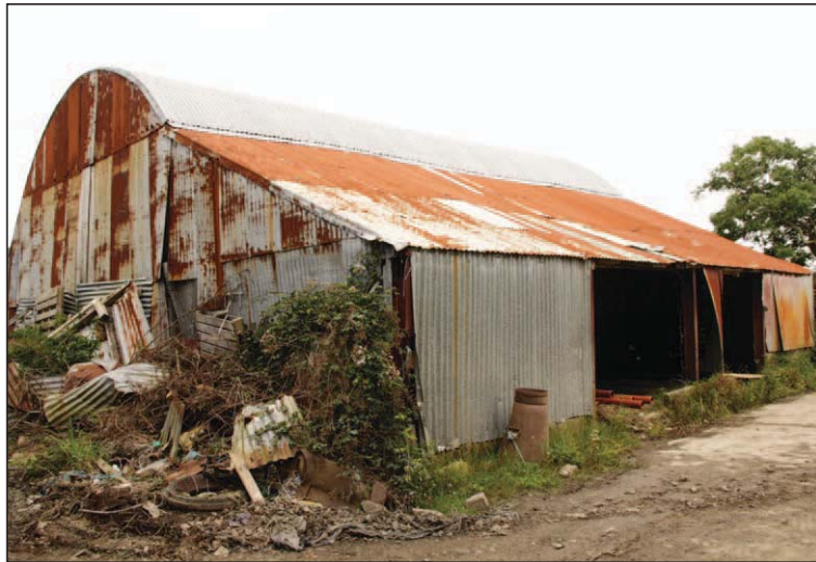
Plate 54 - North and east elevations B06
