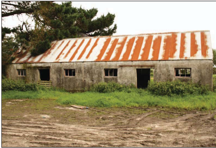
Plate 26 - Southwest elevation A07
