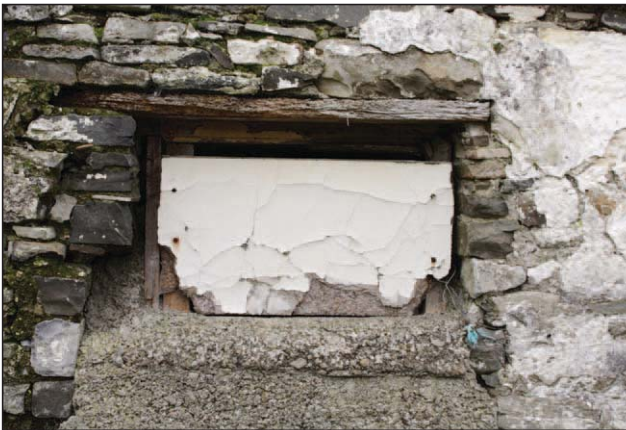
Plate 4 - Window opening southeast elevation A01
