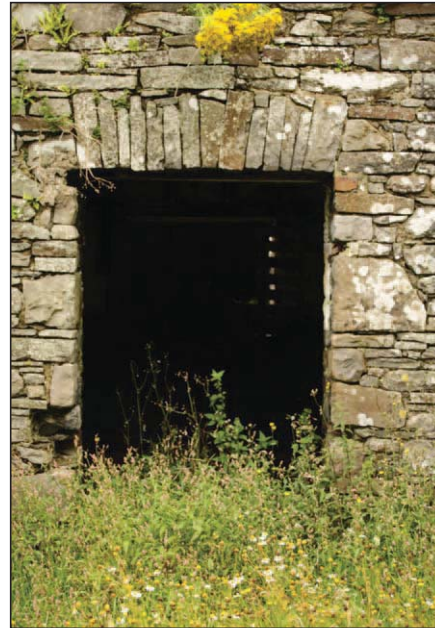
Plate 47 - Door opening west elevation B03
