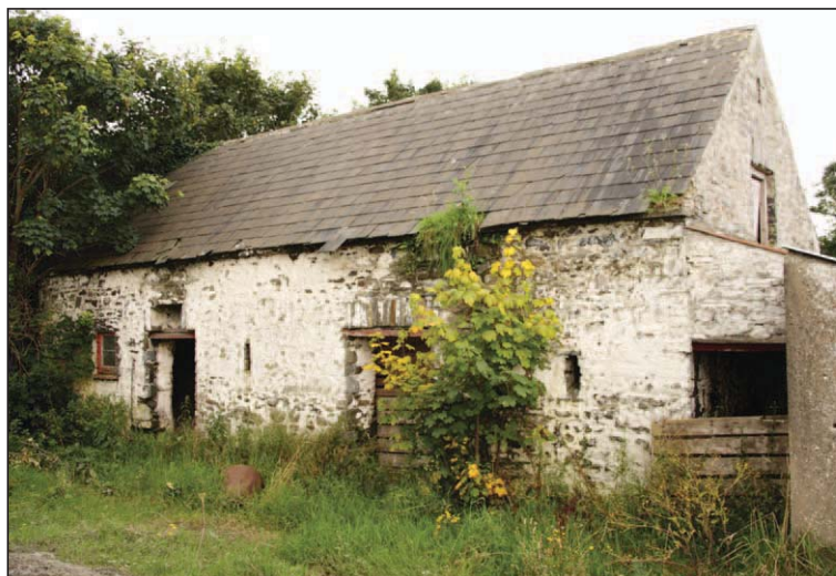
Plate 43 - East and north elevations B03
