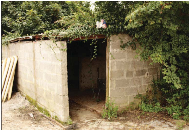
Plate 55 - North and east elevations B07
