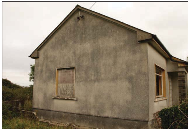
Plate 10 - Southwest elevation A02
