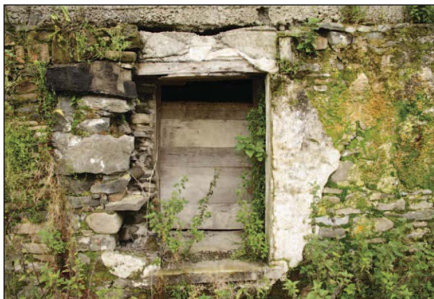
Plate 6 - Window opening to southeast elevation A01
