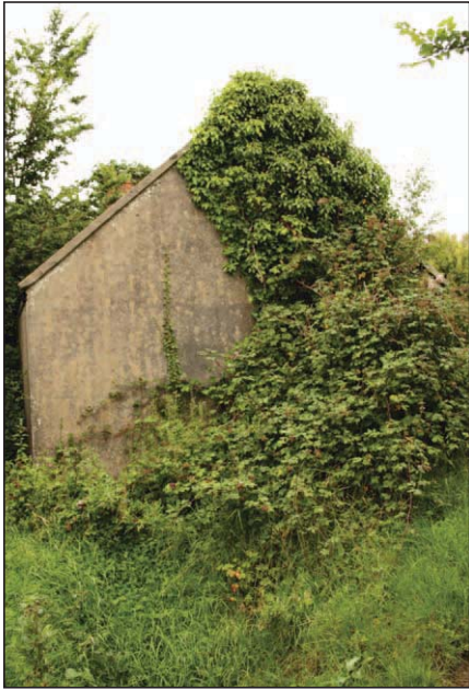
Plate 57 - Southwest elevation C01
