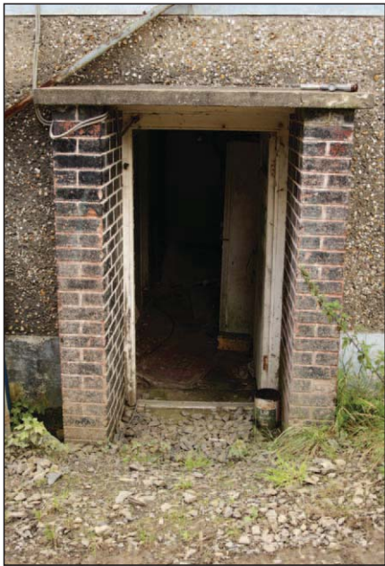
Plate 35 - Door opening west elevation B01
