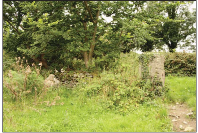
Plate 65 - Boundary wall facing north C05
