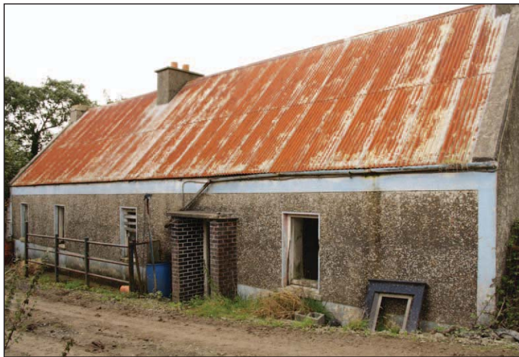
Plate 32 - West elevation B01
