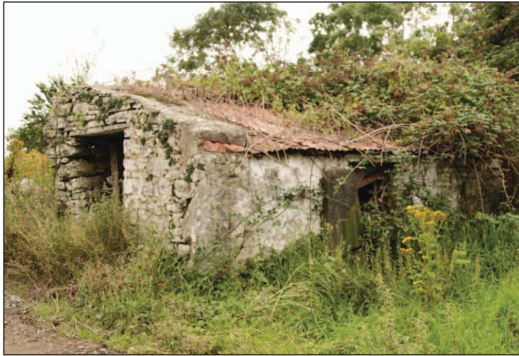
Plate 52 - North and east elevations B04
