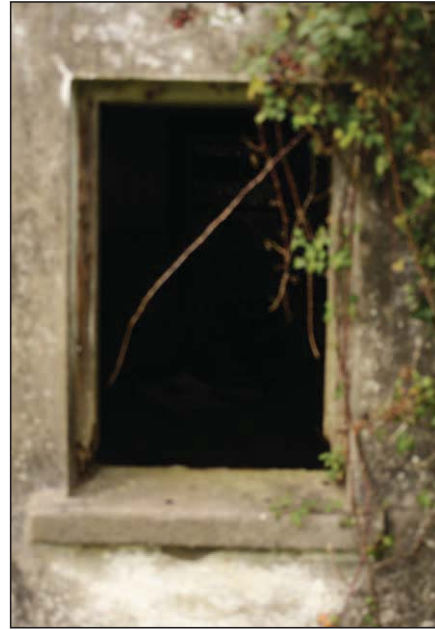
Plate 58 - Window opening southwest elevation C01
