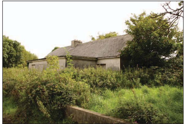
Plate 14 - Northwest and southwest elevations A04
